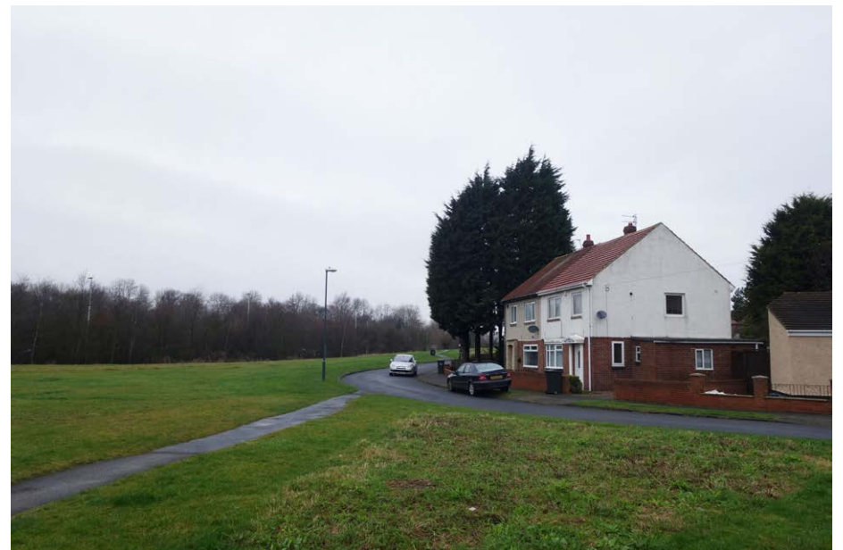
View towards the existing houses on Salcombe Avenue.
