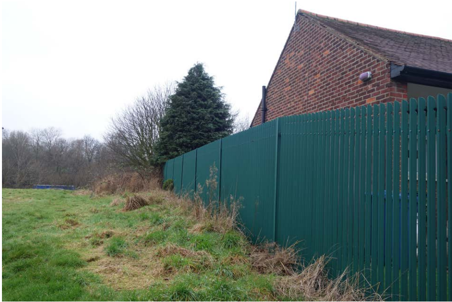
View of the existing boundary to the bungalow at the north of the site.
