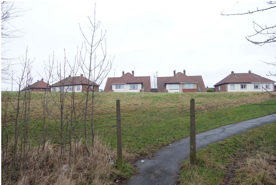
View from the base of the path looking back up towards the development site.
